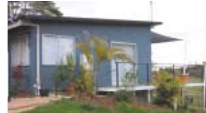
A Skillion Roof House with deck by Unique Structural Company.
