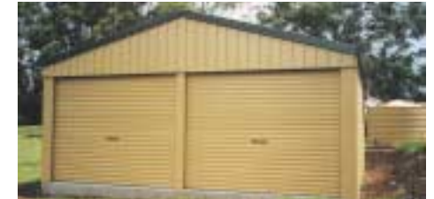
A Unique double garage and Clarke Water Tank. It's all under the one roof.
